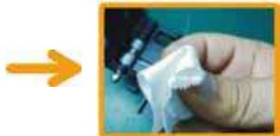
Please ensure that stripped fiber is clean. All objects like coating residue have been removed.
